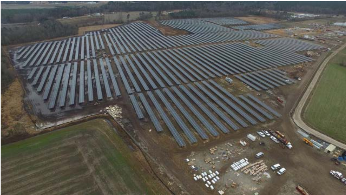
Vivo's North Carolina solar project.
